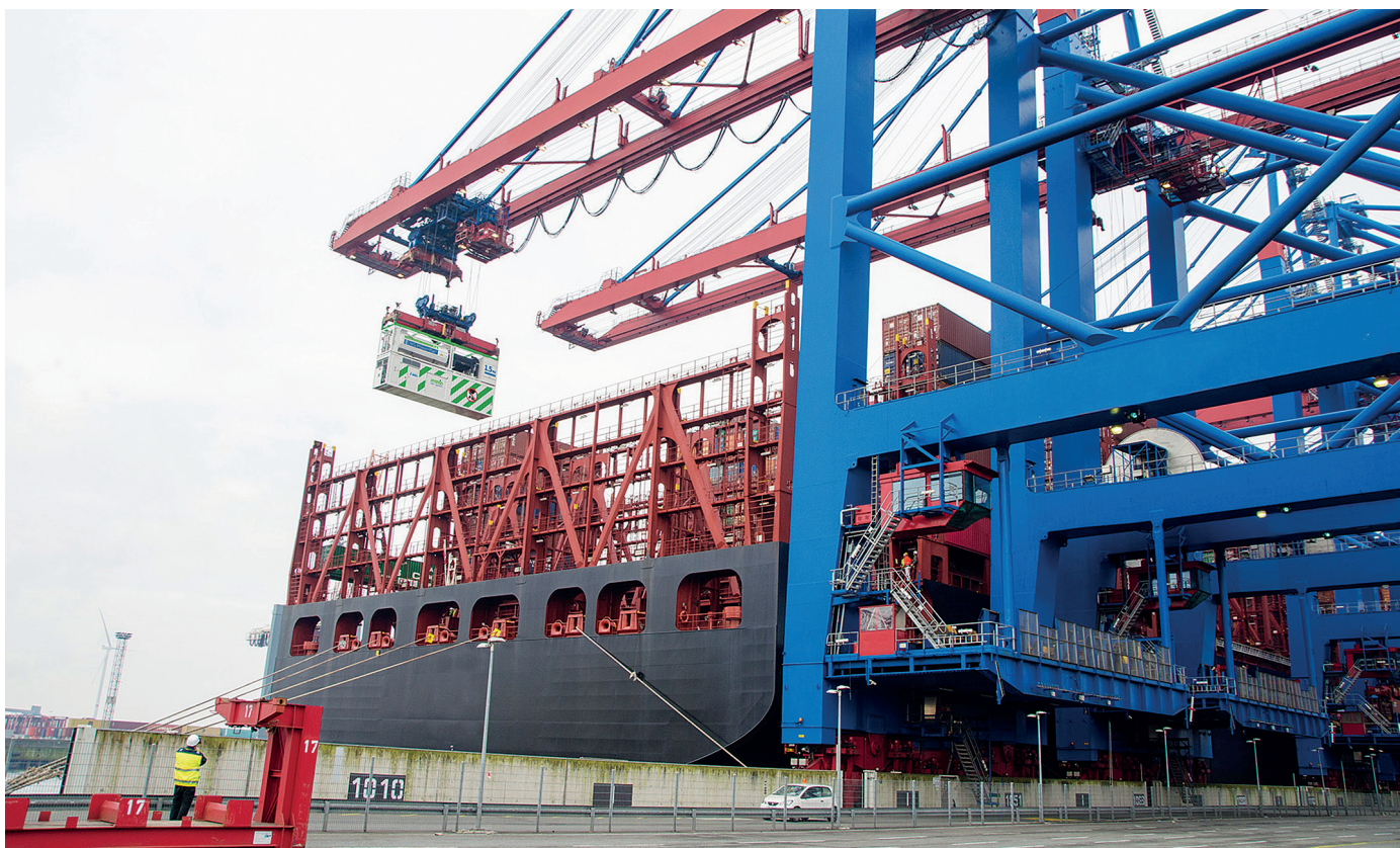
The LNG PowerPac® is lifted onto the rear of the container giant and produces electricity there
